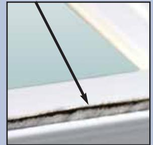
Special double weather stripping seals out drafts and dust and improves insulation.
